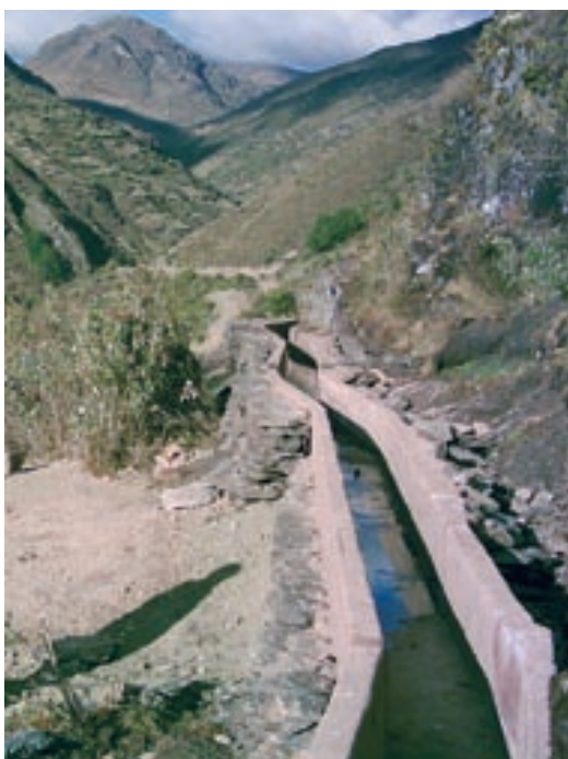
Lifeline: a 14-kilometre canal through this barren region was required.
